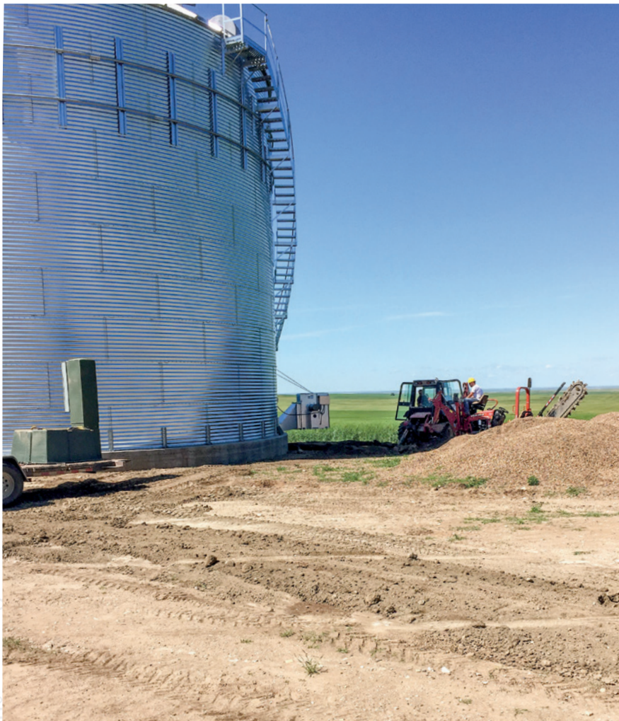
A construction task being completed for grain bins.
